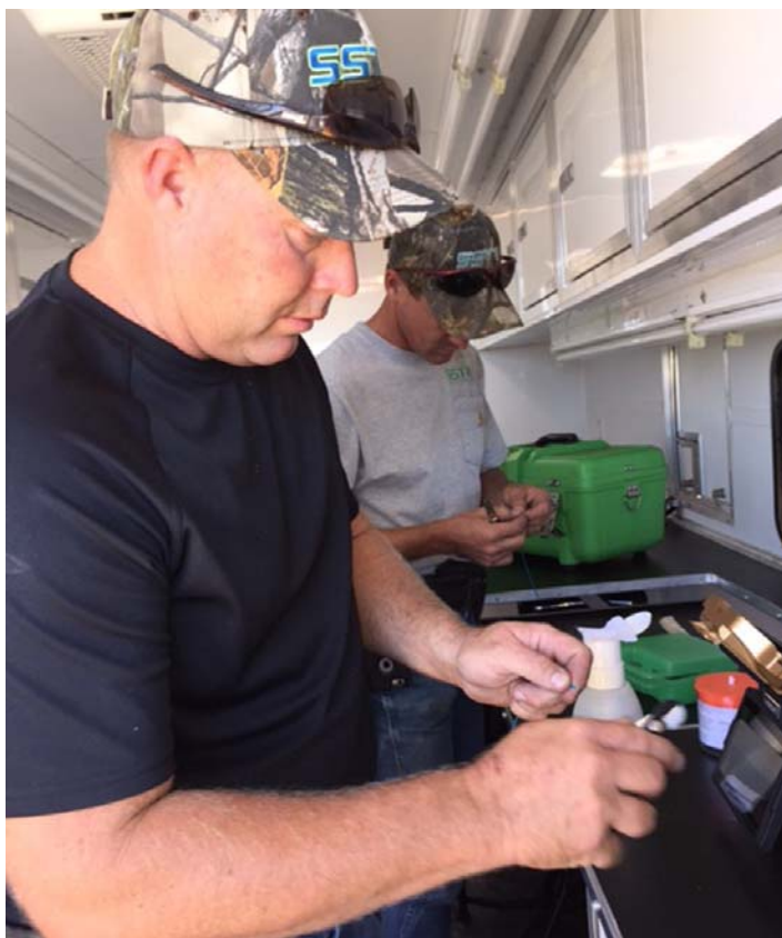
SST AT WORK. . . Scott Tye, left, and Brad Hokit, work inside SST's fiber trailer stripping the ends of fiber cables. Tiny glass strands within the cables are placed into specialized equipment where heat fuses the ends together.
